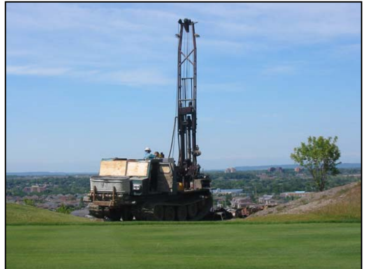
Drilling landfill gas wells in the closed Britannia Sanitary Landfill Site (BraeBen Golf Course)
