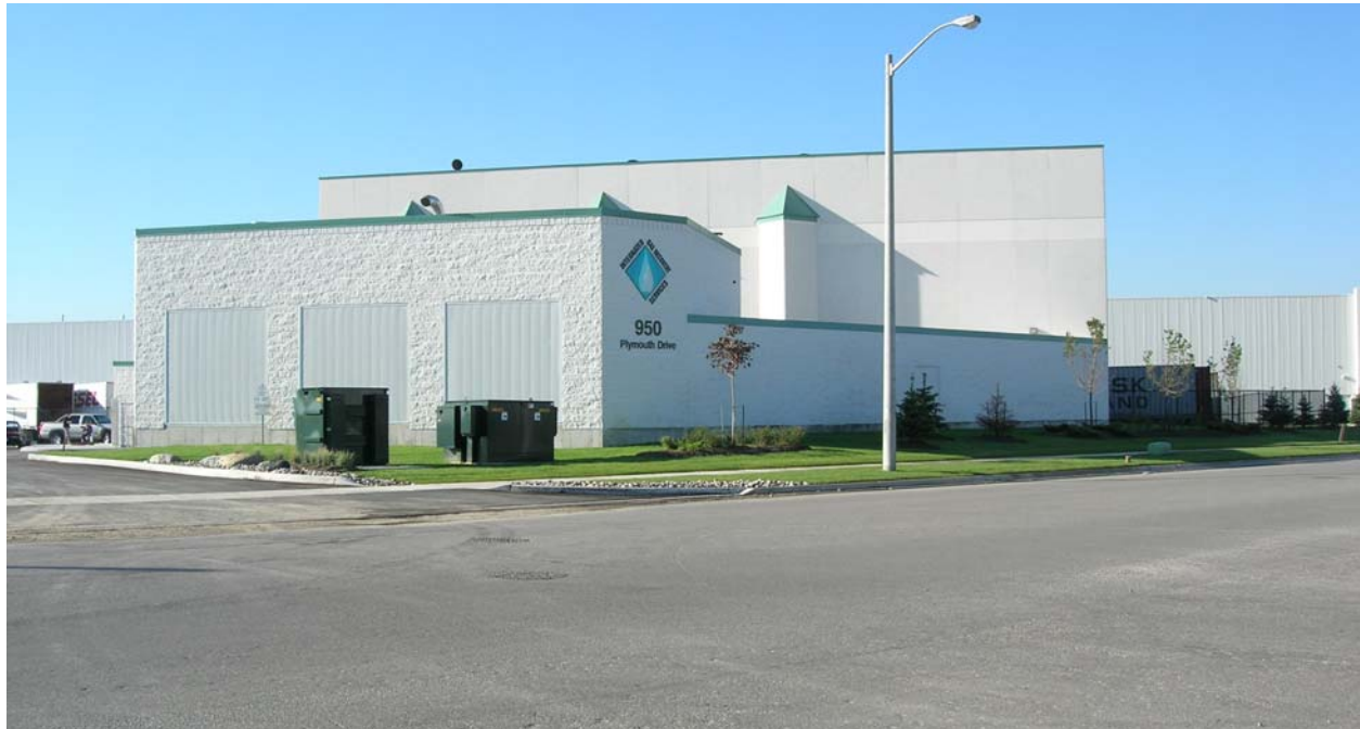
Britannia Landfill Gas Compression and Electrical Generation Facility
