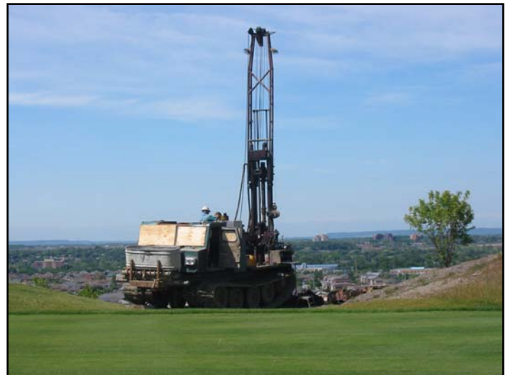
Drilling landfill gas wells in the closed Britannia Sanitary Landfill Site (BraeBen Golf Course)
