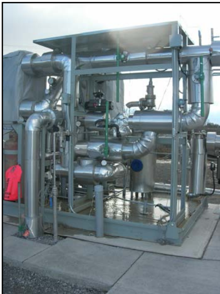
Gas Dryer Skid at the East Landfill Facility
